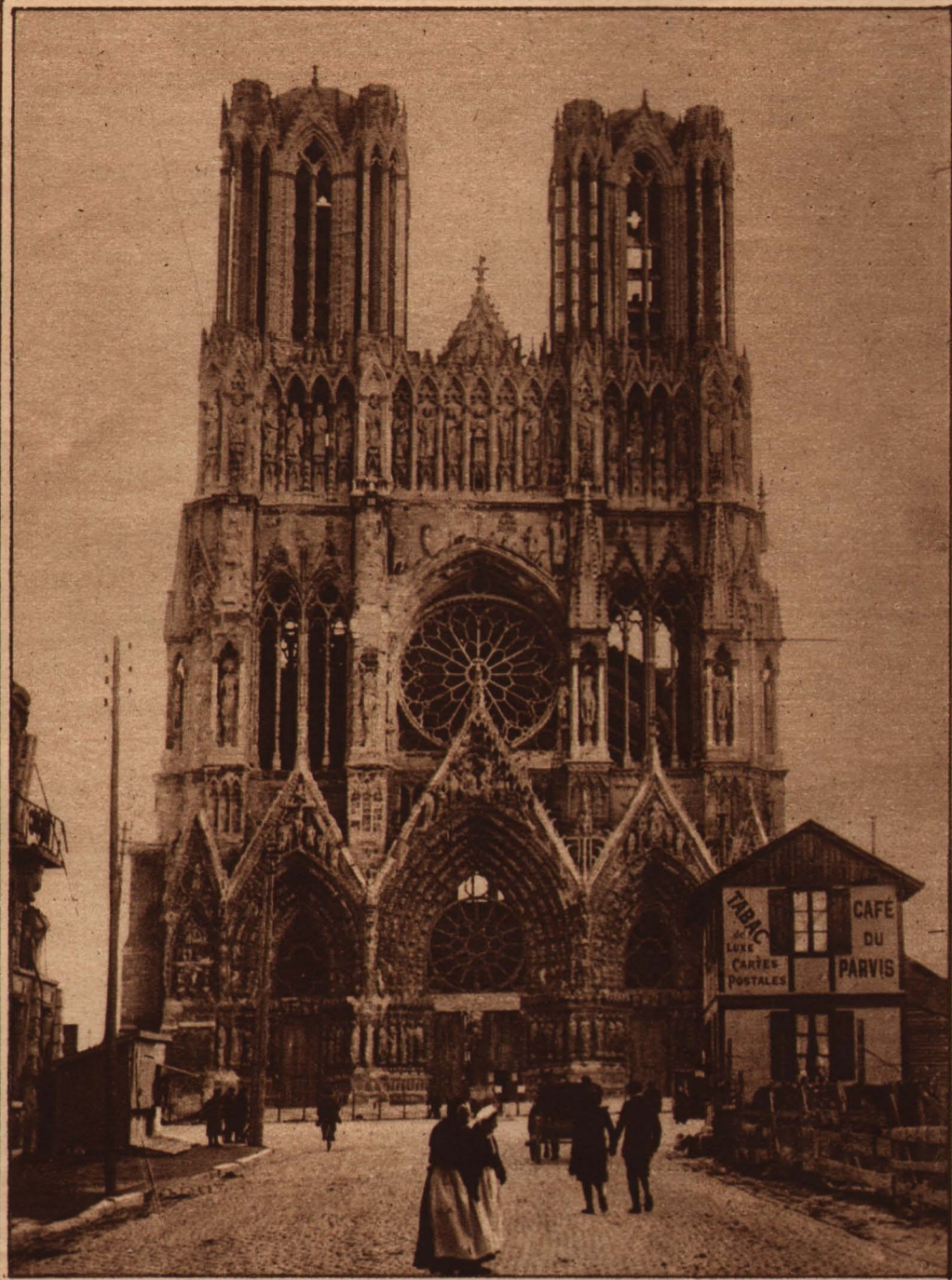
Rheims Cathedral as it looks today, while the work of restoration is being carried on. The ravages suffered by the famous building during the war are being rapidly made good by skilled workmen under the supervision of the greatest architects in France.
