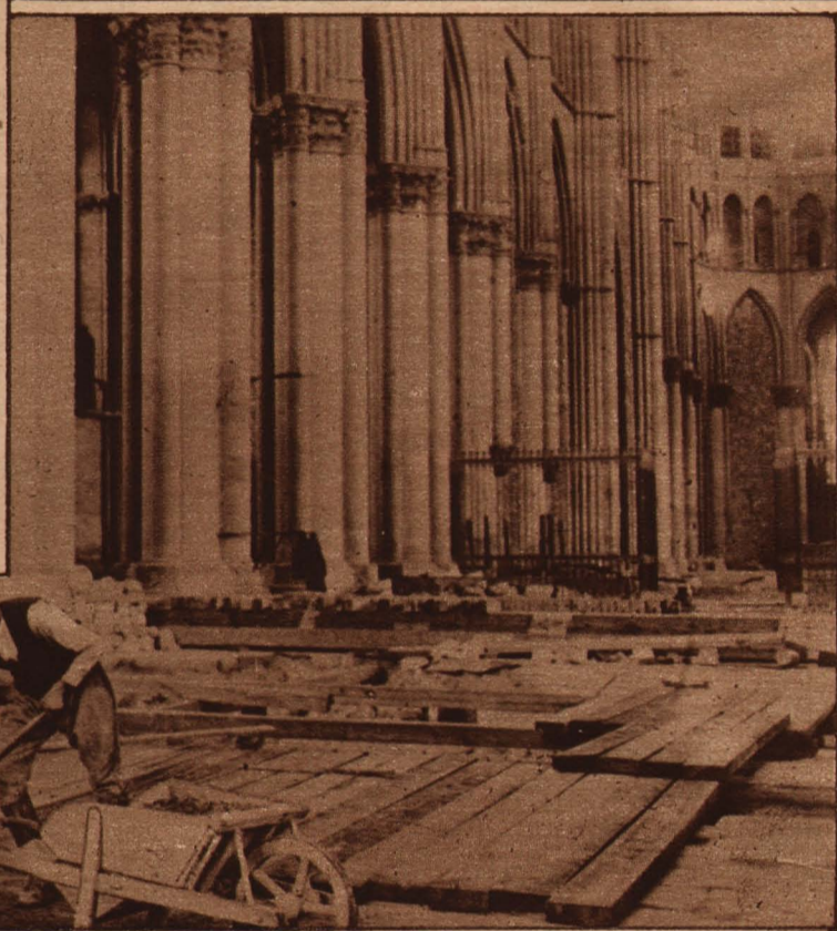
Interior scene, showing workman removing debris. The new columns that have been put in place of those shattered by gun fire are in evidence. While some of the damage done during the siege is irreparable, most of it can be made good.
