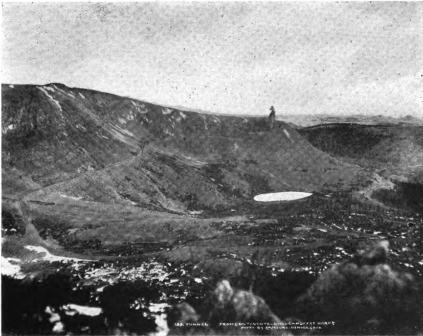
Another View of the Continental Divide, with Train about to enter Tunnel 32 of the "Moffat Road."
