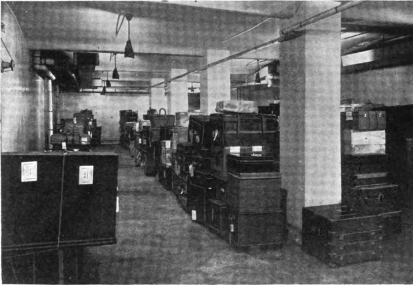
Storage Vault for Valuables, Germantown Trust Co., Philadelphia.
