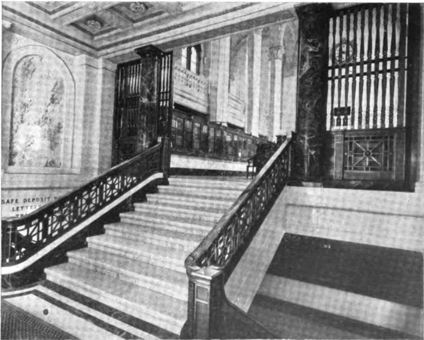
A Glimpse of the Main Banking Room as seen from the Vestibule. At the extreme left the stair turns down to the Safe Deposit Vaults.
