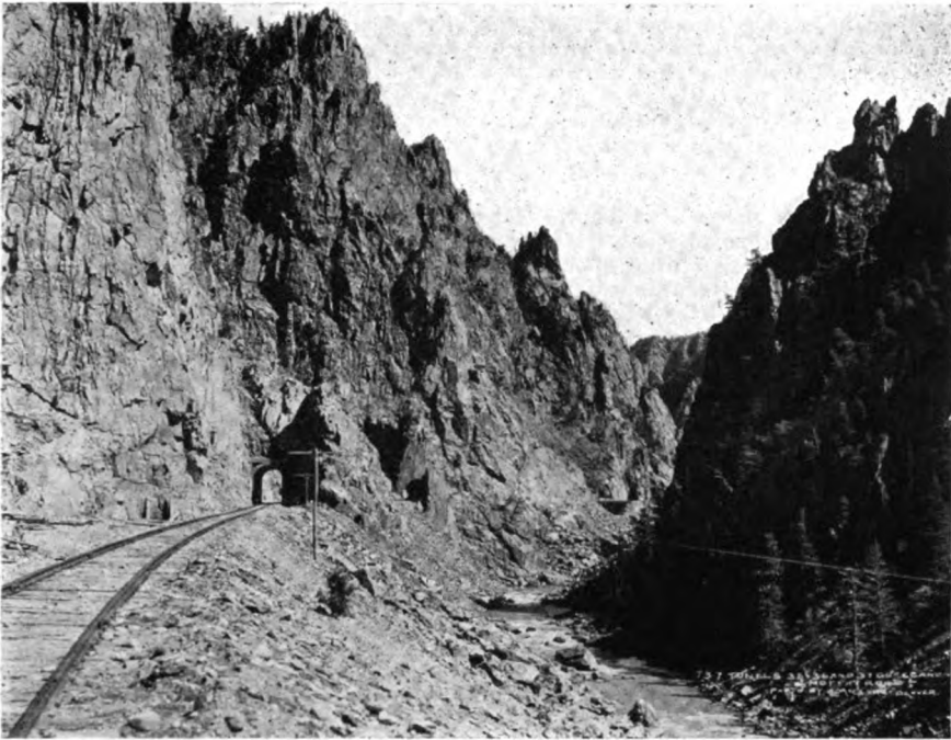
Some of the Tunnels through which Passengers on the Denver, Northwestern and Pacific Road are taken.
