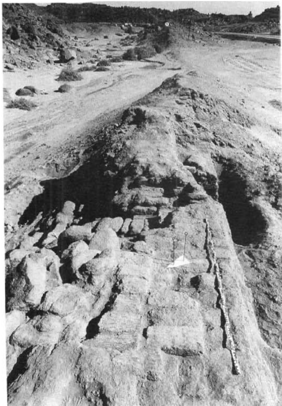
b) The wall at the western foot of Gebel el-Granite (site X) showing destruction by water and repeated repairs
