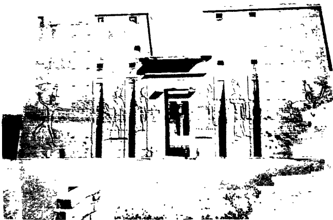
PYLON OF THE TEMPLE OF IDJU
