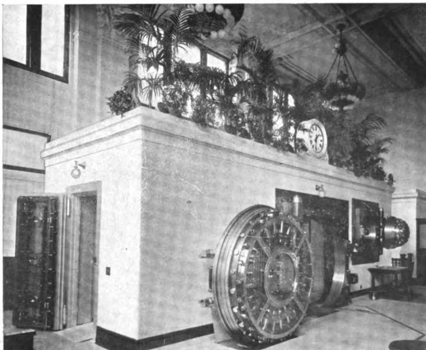
VAULT IN THE SAVANNAH BANK AND TRUST COMPANY, SAVANNAH, GA.
