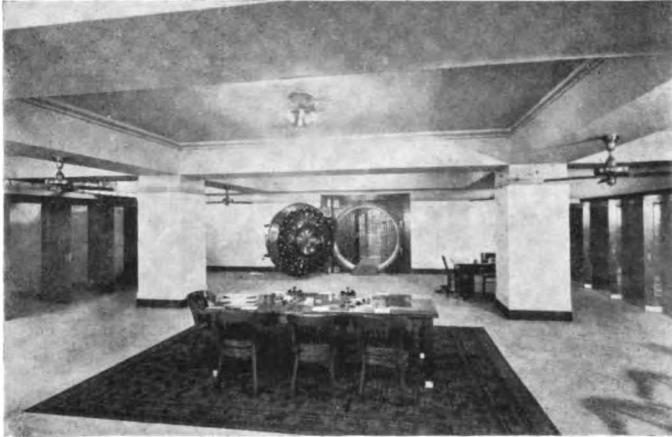
LOBBY TO SAFE DEPOSIT DEPARTMENT
