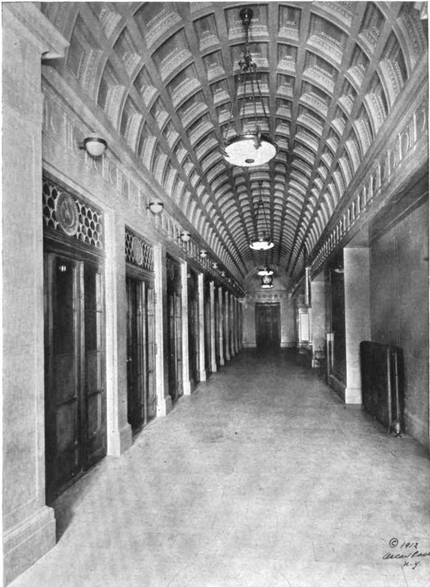
ELEVATOR CORRIDOR, ENTRANCE TO OFFICES FROM 14 WALL STREET, BANKERS TRUST COMPANY BUILDING, NEW YORK
