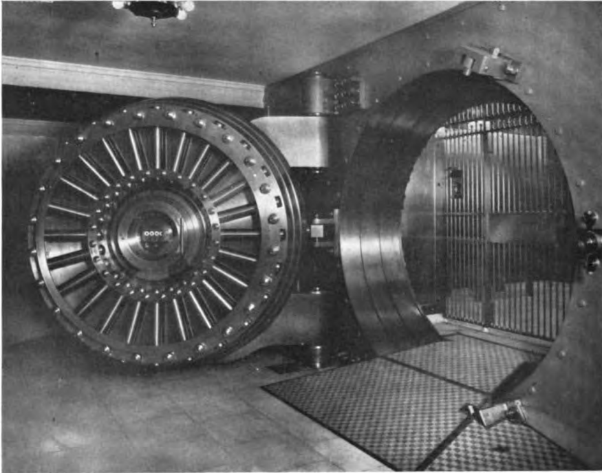
MAMMOTH VAULT DOOR OPEN, SHOWING BOLT WORK ESSEX COUNTY NATIONAL BANK, NEWARK, N. J.
