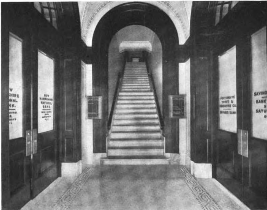
ENTRANCE TO THE BANKING ROOMS IN THE NEW HAMPSHIRE NATIONAL BANK, PORTSMOUTH
