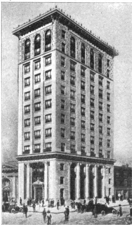
NEW BANK AND OFFICE BUILDING IN COURSE OF CONSTRUCTION FOR THE CITIZENS NATIONAL BANK, RALEIGH, N. C.
