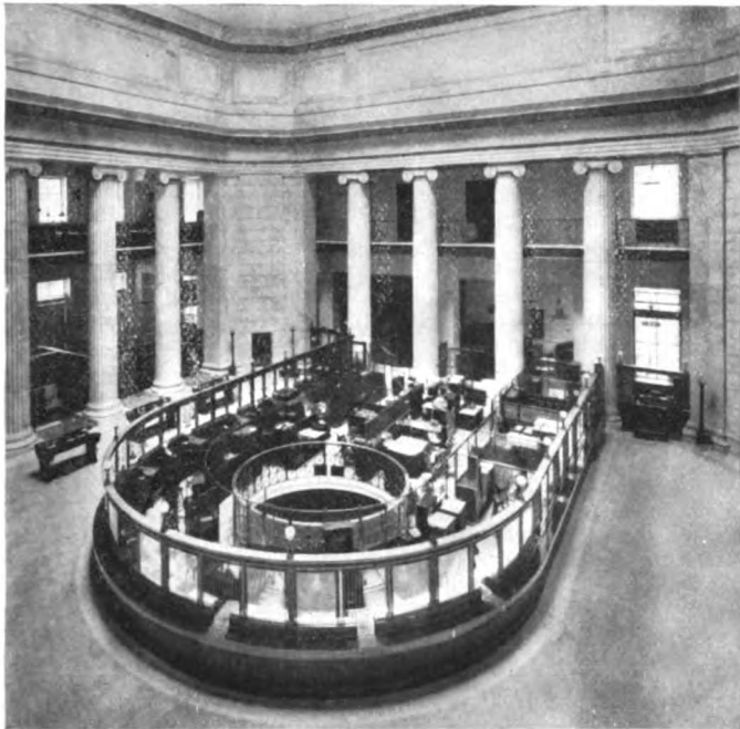
VIEW OF MAIN BANKING ROOM GIRARD TRUST COMPANY, PHILADELPHIA
