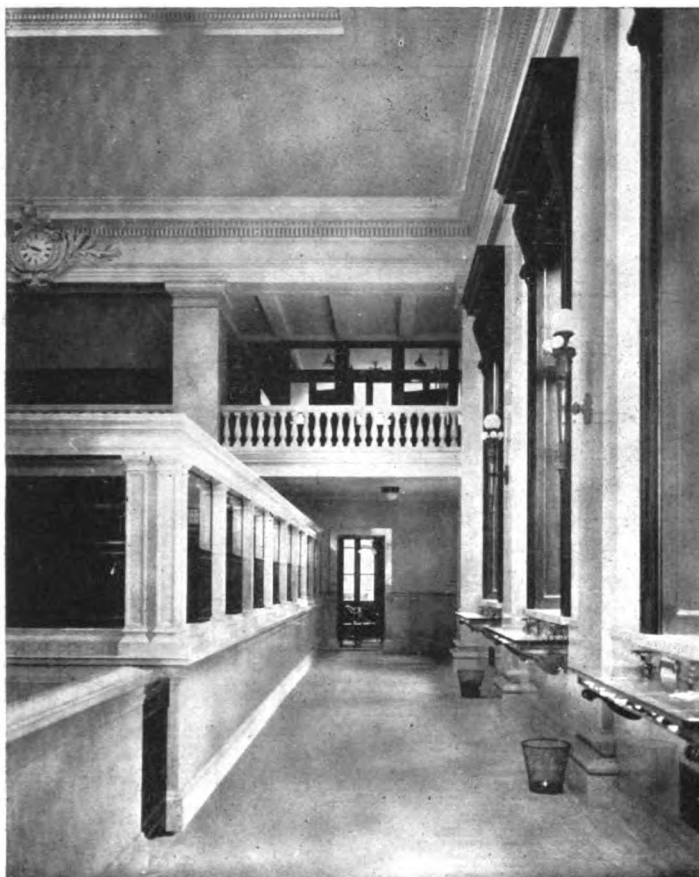
BARNETT NATIONAL BANK, JACKSONVILLE, FLA. EASTERN LOBBY, LOOKING NORTH.
