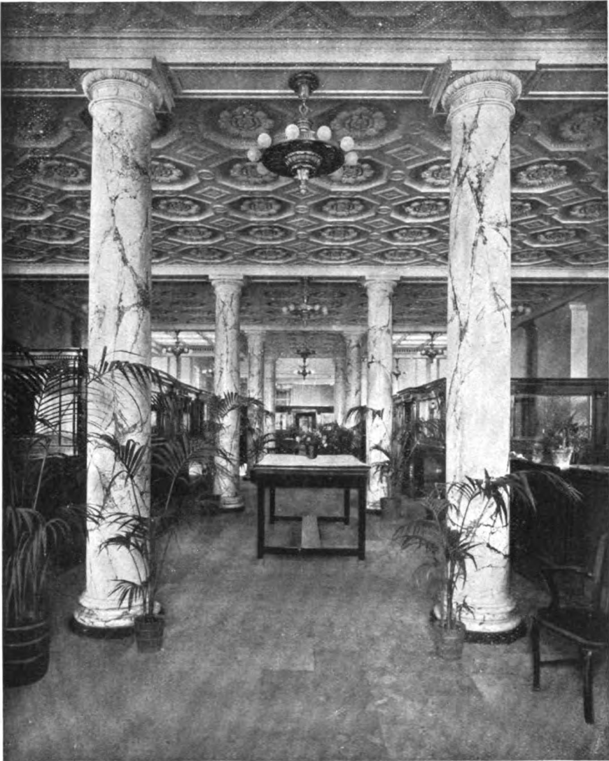
A VIEW IN THE MAIN BANKING ROOM, NATIONAL STATE AND CITY BANK, RICHMOND, VA.
