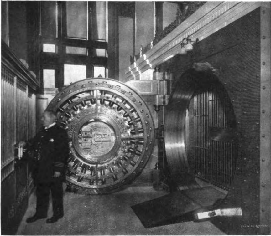
SAFETY VAULT DOOR
