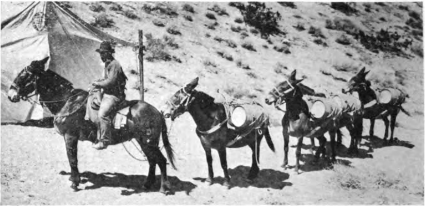
AT THE OUTLET, MANY MILES OF THE AQUEDUCT ZONE WERE INACCESSIBLE. IN THE CONSTRUCTION OF ROADS THESE SURL-LOADED BEASTS OF BURDEN WERE EMPLOYED TO CARRY WATER, PROVISIONS AND DYNAMITE FOR BLASTING, AS SHOWN IN THE ILLUSTRATION.
