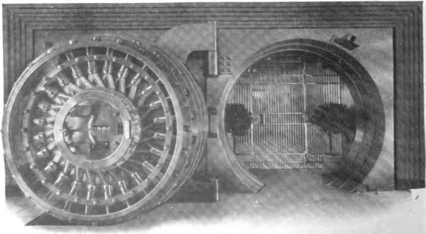
VESTIBULE OF SAFE DEPOSIT VAULT, SHOWING FIFTY-TON DOOR
