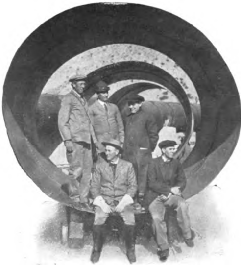
LOS ANGELES AQUEDUCT—A SECTION OF ONE OF THE GREAT STEEL INVERTED SIPHONS, ELEVEN FEET IN DIAMETER, WITH STEEL ONE-QUARTER TO ONE-HALF INCHES IN THICKNESS.
