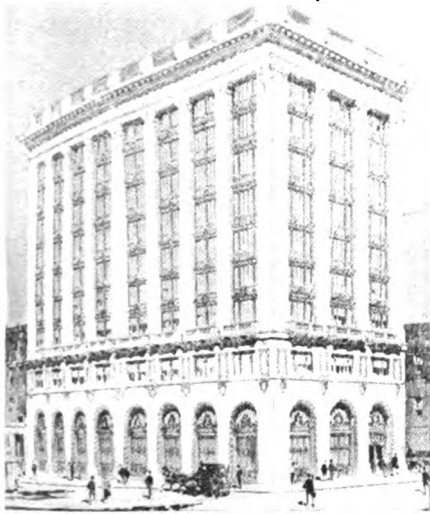
MERCHANTS NATIONAL BANK, STATE STREET. NOW UNDER CONSTRUCTION
