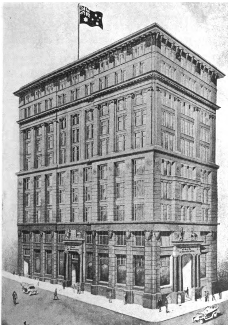
HEAD OFFICE BUILDING OF THE COMMONWEALTH BANK NOW IN COURSE OF CONSTRUCTION AT SYDNEY, N. S. W.
