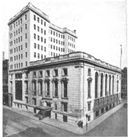
FIRST NATIONAL BANK, FEDERAL STREET
