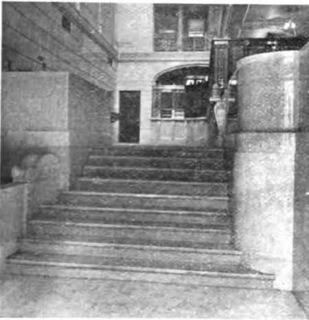
APPROACH TO BANKING FLOOR
