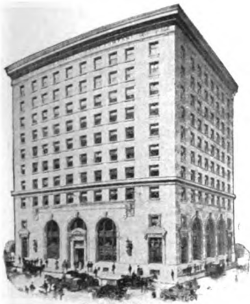
BOSTON SAFE DEPOSIT AND TRUST CO., FRANKLIN STREET
