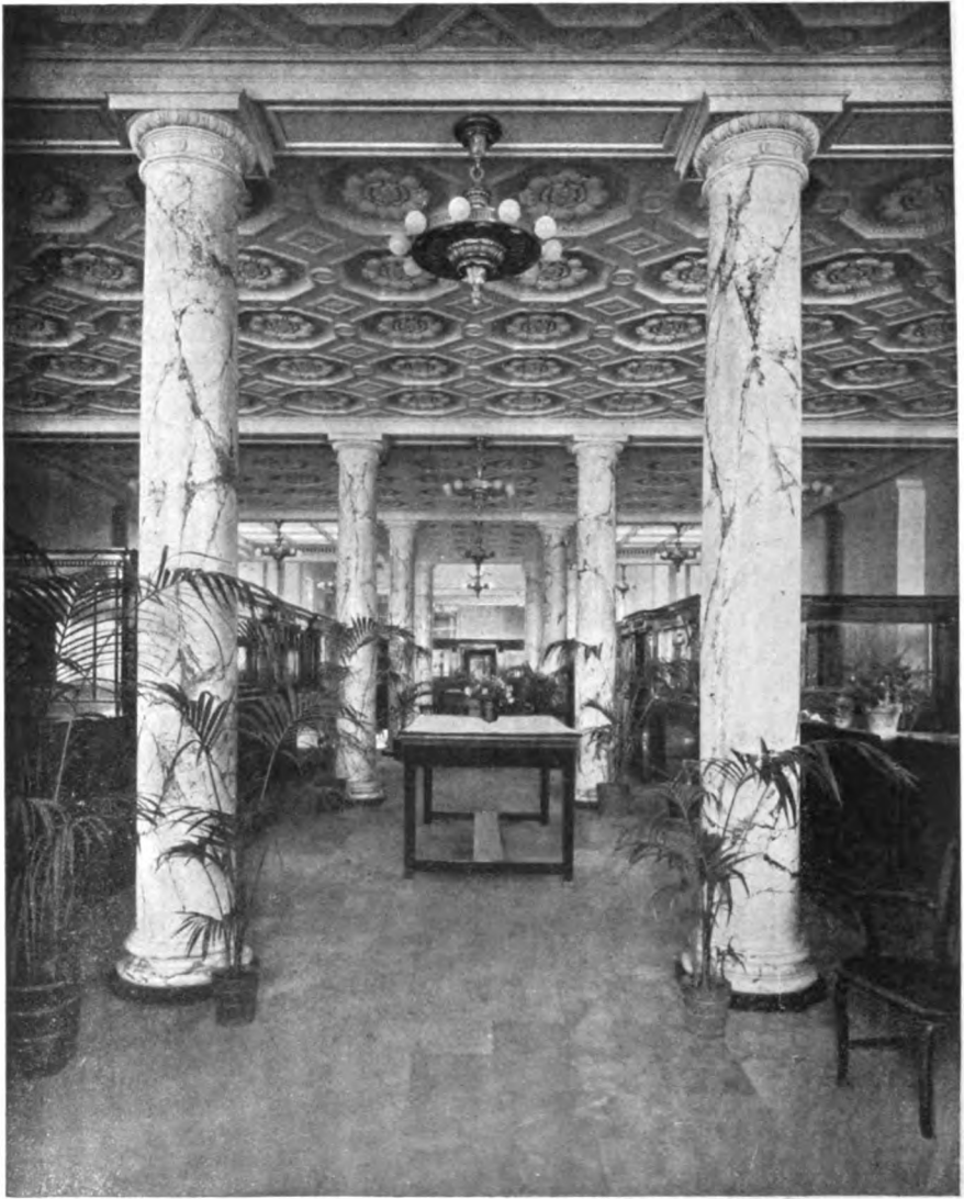
MAIN BANKING ROOM, NATIONAL STATE AND CITY BANK, RICHMOND
