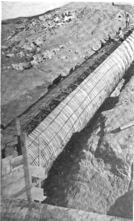
BUILDING THE ELSMERE CONCRETE SIPHON
