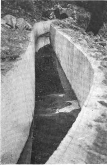
CONCRETE INTAKE DITCH LEADING TO UPPER END OF TUNNEL NO. 1
