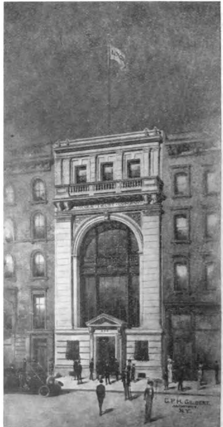
BUILDING OF THE LINCOLN TRUST COMPANY, NEW YORK, IN COURSE OF CONSTRUCTION.
