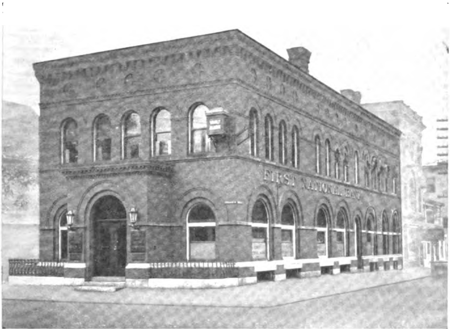
FIRST NATIONAL BANK, WHITE RIVER JUNCTION, VERMONT
