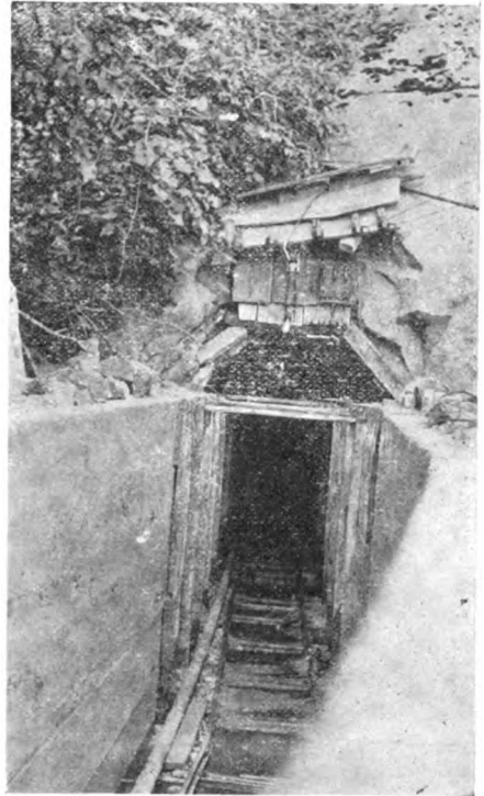
LOOKING THROUGH TUNNEL NO. 11, WHICH IS 1900 FEET LONG, DRIVEN STRAIGHT THROUGH A MOUNTAIN OF SOLID GRANITE. THE WHITE SPOT IN THE CENTRE OF THE ARCH IS THE PORTAL AND REFLECTION AT THE OPPOSITE END
