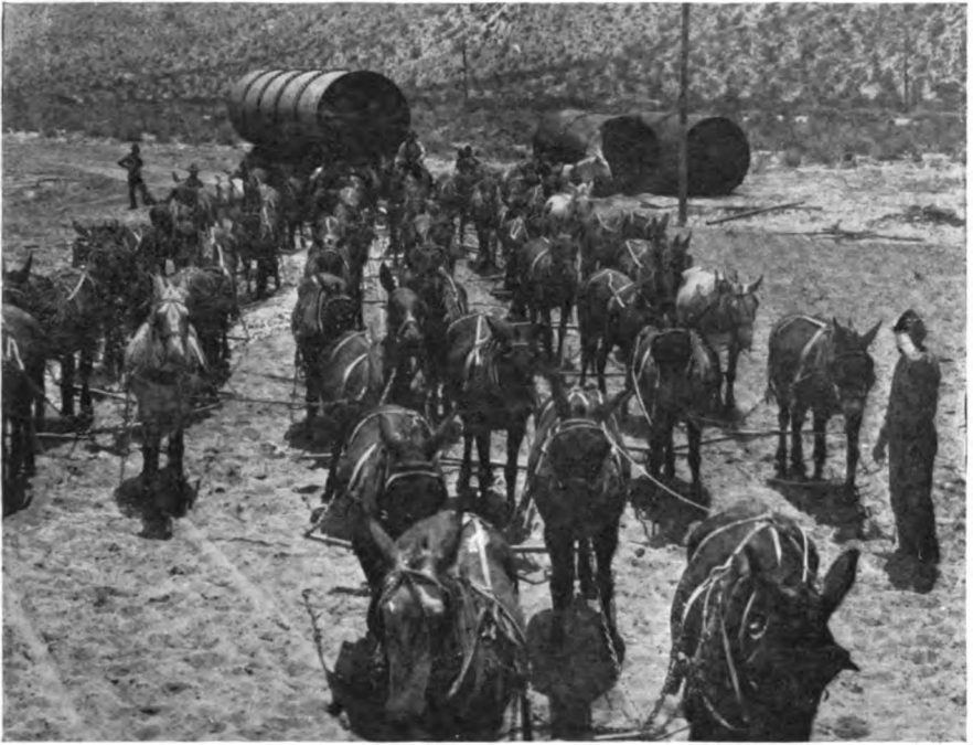
SECTIONS OF THE GREAT SIPHON WERE HAULED FROM THE RAILROAD STATION, SEVEN MILES OVER SANDY ROADS IN SPECIALLY CONSTRUCTED WAGONS DRAWN BY FIFTY HEAD OF MULES.
