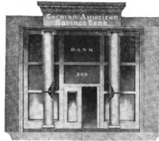
THE GERMAN AMERICAN TRUST AND SAVINGS BANK MOVED TO THIS LOCATION AT 223 SOUTH SPRING STREET, IN 1906. A BRANCH WAS RETAINED AT THE OLD LOCATION AT MAIN AND FIRST STREETS
