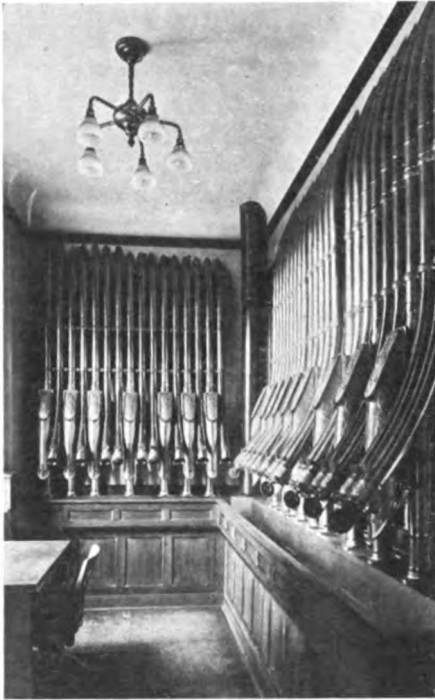
CENTRAL EXCHANGE FOR PNEUMATIC TUBES AND TELEPHONES
