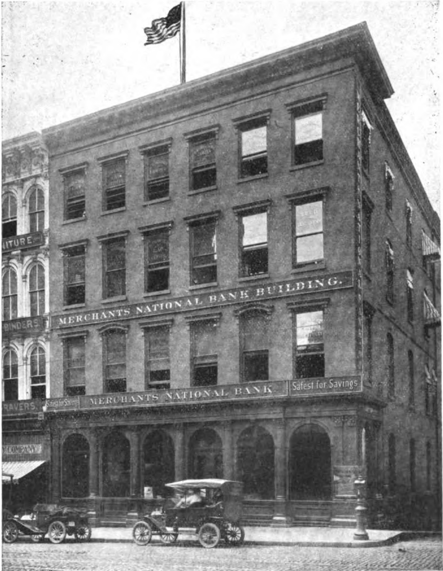
MERCHANTS NATIONAL BANK BUILDING, RICHMOND
