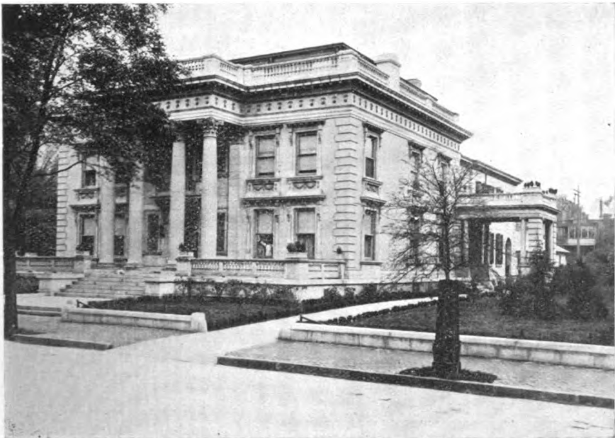
A TYPICAL CITY RESIDENCE
