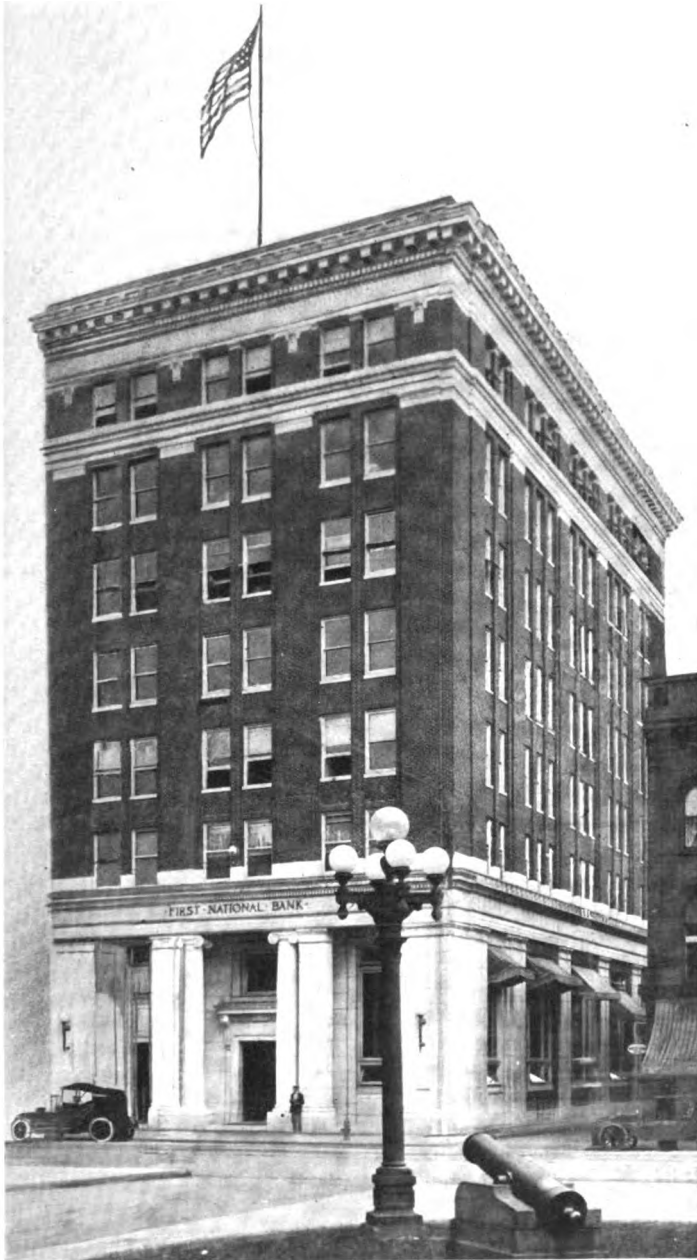
NEW BUILDING FIRST NATIONAL BANK, WILLIAMSPORT, PA.
