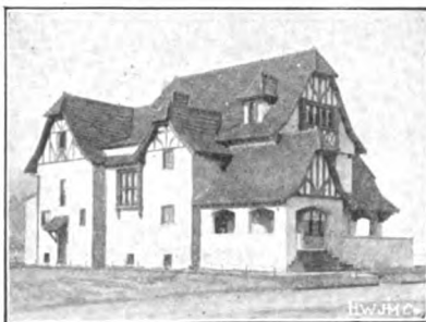
Residence of M. C. Madsen, Long Beach, L. I. Covered with J-M Asbestos Stucco. Kirby, Petit & Green, Architects, New York.
