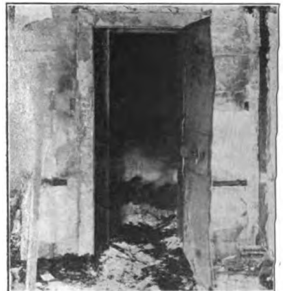
VAULT OF THE BANGOR POST-OFFICE AFTER THE FIRE; EVERYTHING DESTROYED
