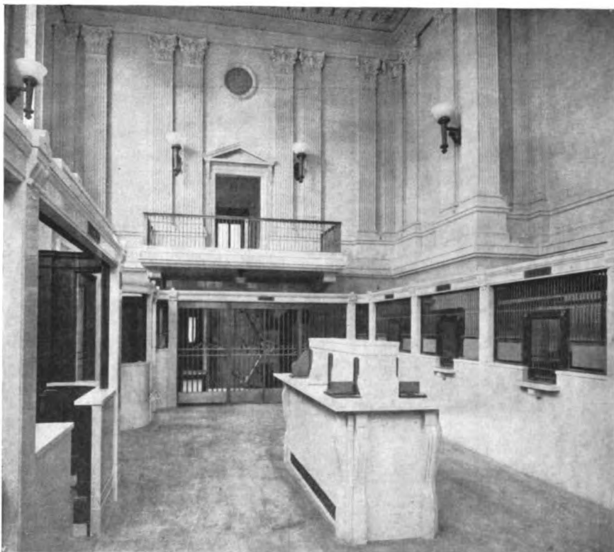
PARTIAL VIEW OF MAIN BANKING ROOM MANSFIELD SAVINGS BANK, MANSFIELD, OHIO
