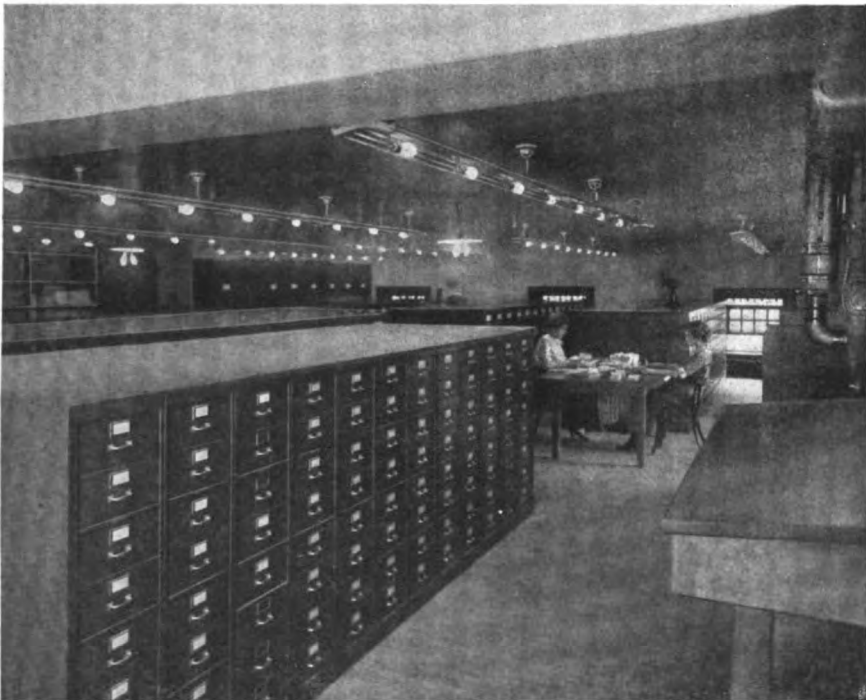
PART OF THE BANK'S FILING ROOM
