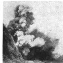
A DYNAMITE BLAST IN CULEBRA CUT
