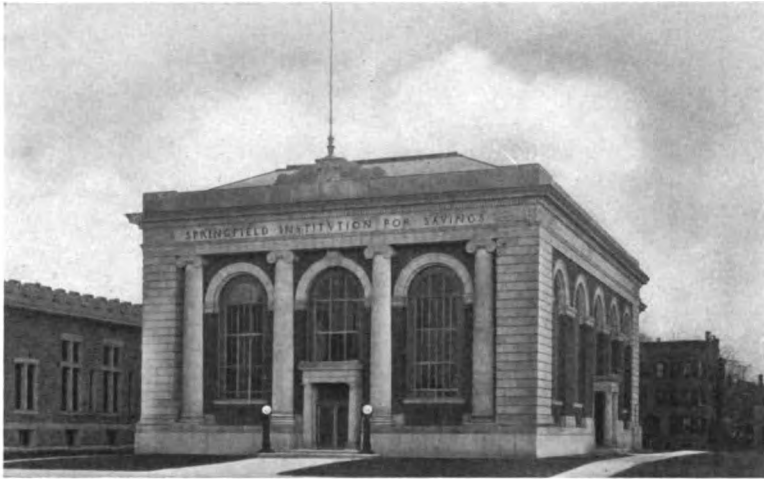
SPRINGFIELD INSTITUTION FOR SAVINGS, SPRINGFIELD, MASS. A GOOD EXAMPLE OF THE EXCLUSIVE TYPE OF BANK BUILDING (Illustration by courtesy of Messrs. Hoggson Bros., N. Y.)
