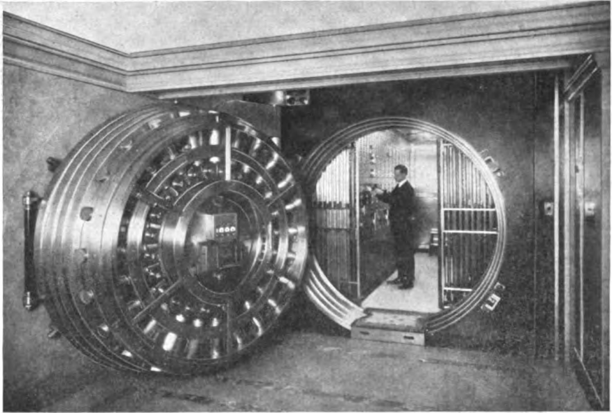
ENTRANCE DOOR TO SAFE-DEPOSIT VAULT
