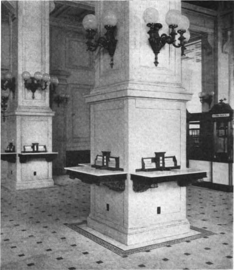
A CORNER, PIERS, LIGHTING FIXTURES, AND MARBLE TOP BRACKET DESKS FOR CUSTOMERS
