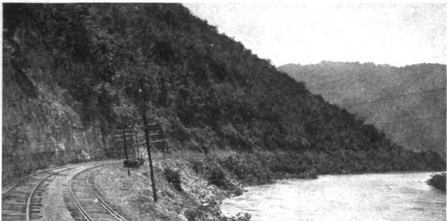
C. & O. RAILWAY DOUBLE TRACK ON NEW RIVER, WEST VIRGINIA
