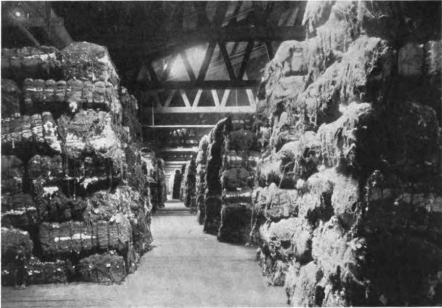
COTTON STORAGE ON SECTION OF AMERICAN DOCK PIERS, SHOWING SPACE OCCUPIED BY 6,000 BALES, ALL PROTECTED BY AUTOMATIC SPRINKLERS
