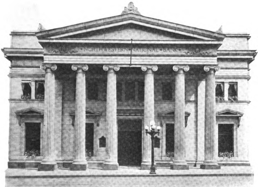
NORTHWESTERN NATIONAL BANK, MINNEAPOLIS, MINN.
