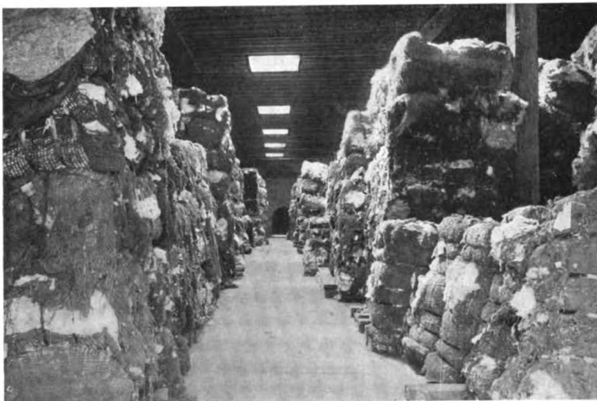
COTTON STORAGE IN AMERICAN DOCK STORE, SHOWING COMPARTMENT HOLDING 4,000 BALES, ALL PROTECTED BY AUTOMATIC SPRINKLERS
