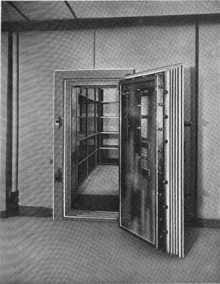
ONE OF THE STORAGE VAULTS FIRST NATIONAL BANK, SYRACUSE, N. Y.
