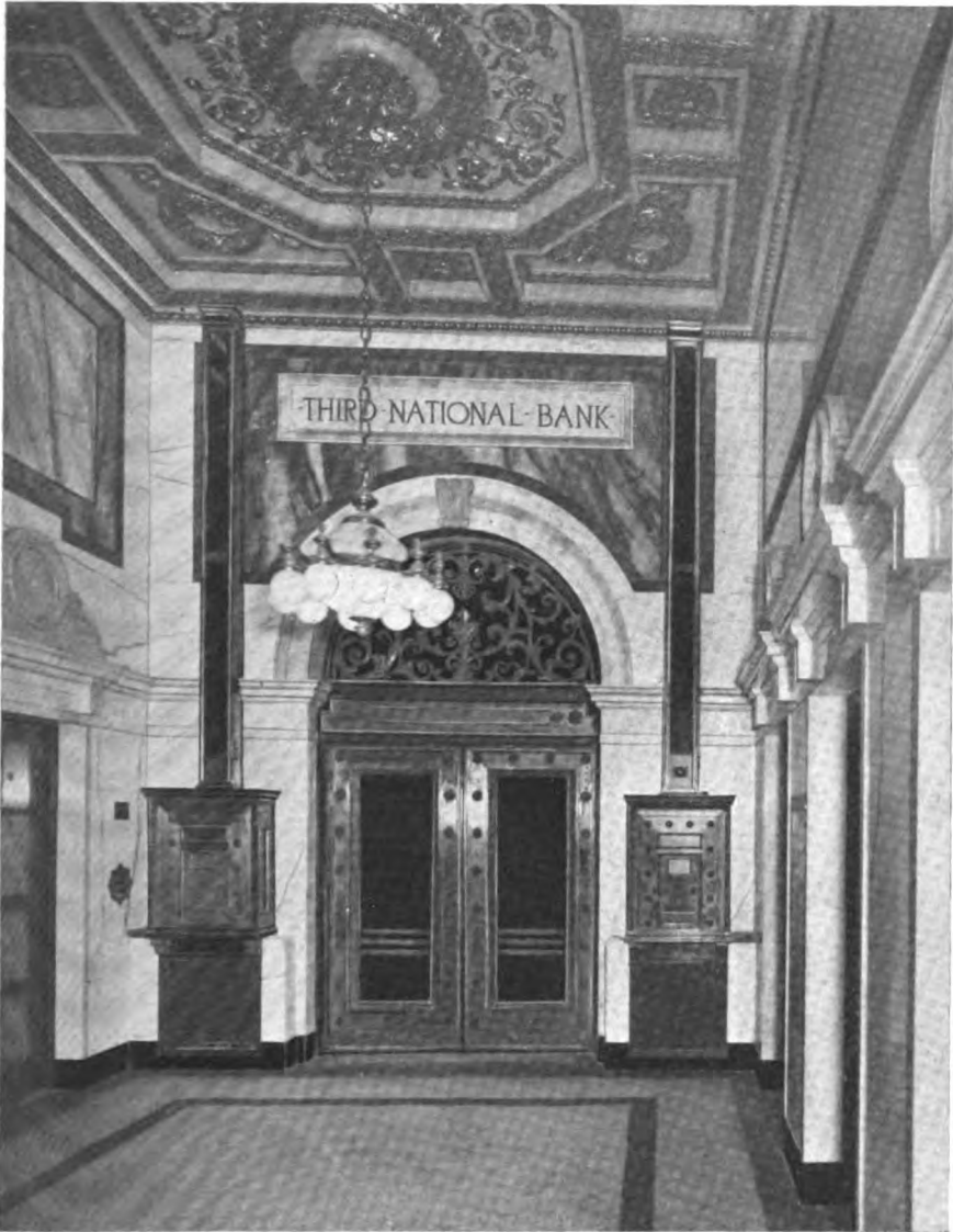
ELEVATORS AND ENTRANCE TO BUILDING
