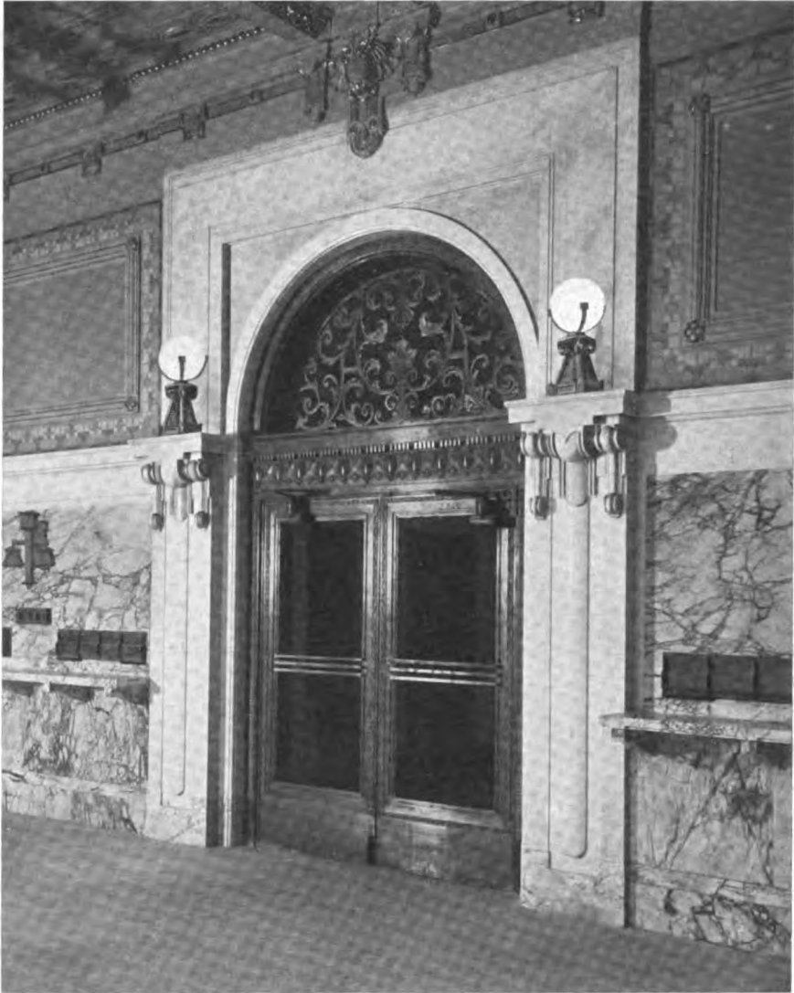
OLIVE STREET ENTRANCE (INTERIOR)
