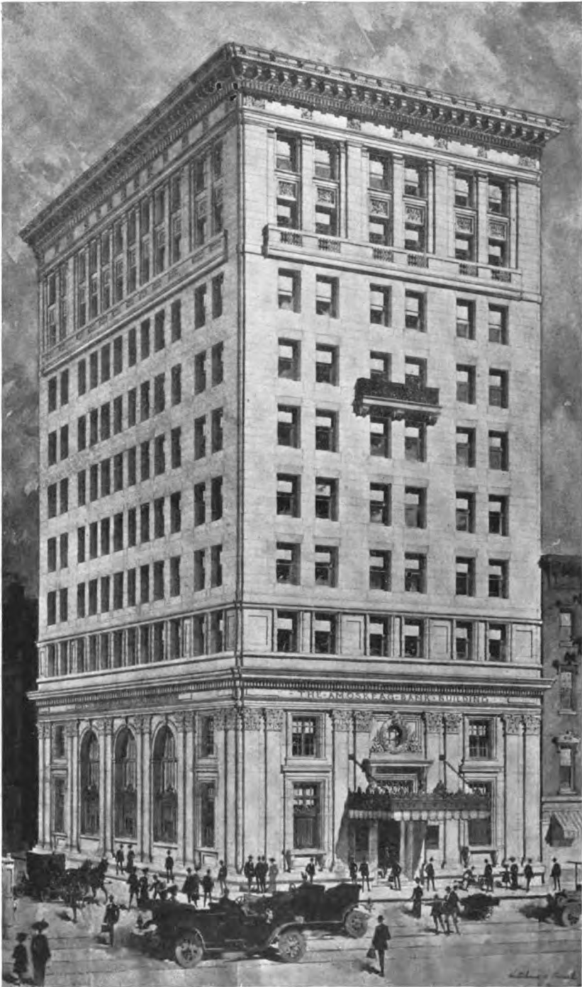
THE AMOSKEAG BANK BUILDING, MANCHESTER, NEW HAMPSHIRE
