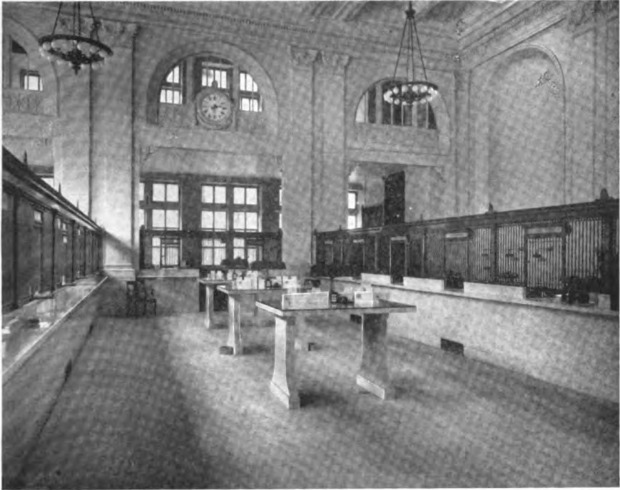
MAIN BANKING ROOM, LOOKING TO THE REAR
