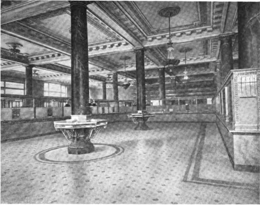
MAIN BANKING ROOM—FROM LOCUST STREET ENTRANCE
