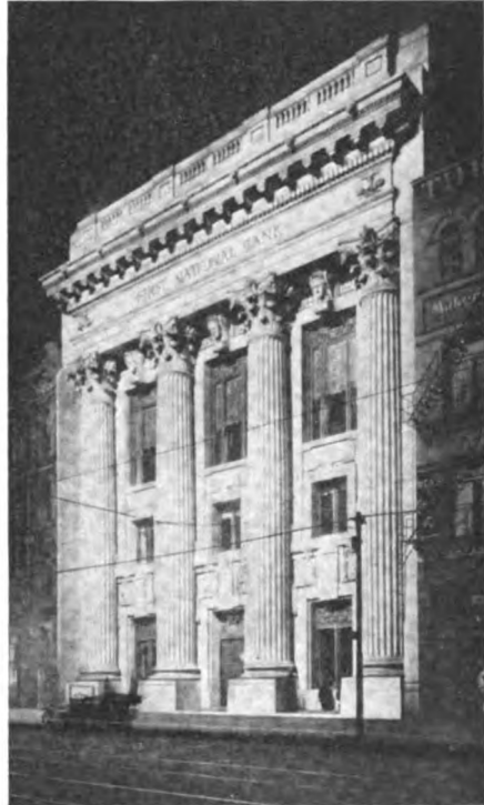
MIDNIGHT ILLUMINATION OF THE BUILDING OF THE FIRST NATIONAL BANK, CLEVELAND
