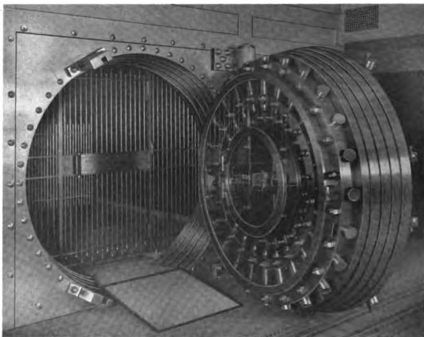
ANOTHER VIEW OF THE MAIN DOOR TO THE VAULTS OF THE NEW YORK COUNTY NATIONAL BANK—DOOR IS HALF CLOSED
