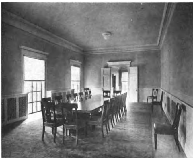
DIRECTORS' ROOM THE NEW HAVEN BANK, N. B. A., NEW HAVEN, CONN.
