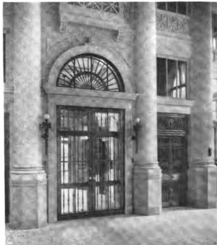
ENTRANCE TO MAIN BANKING ROOM
