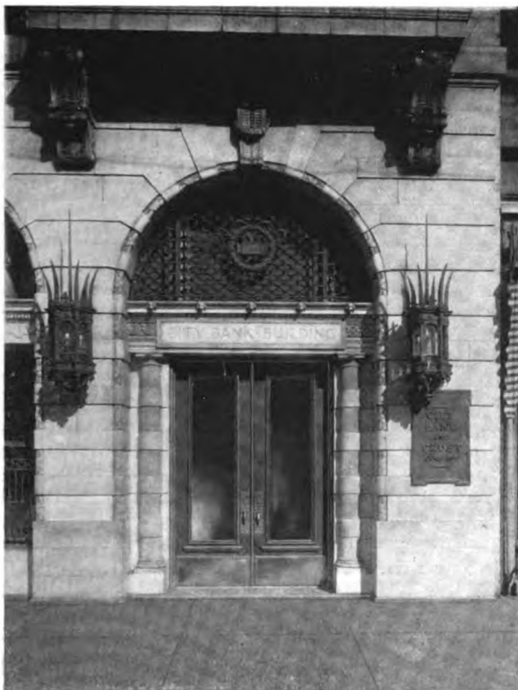
ST. JOSEPH STREET ENTRANCE NATIONAL CITY BANK, MOBILE, ALA.
